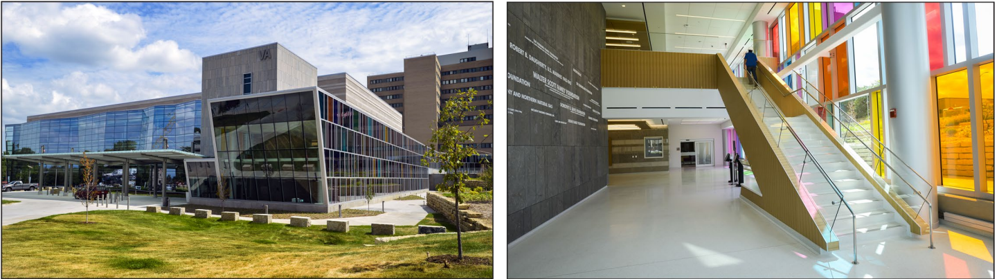
Figure 1: Department of Veterans Affairs' (VA) Ambulatory Care Center in Omaha, NE—Exterior and Interior Views
