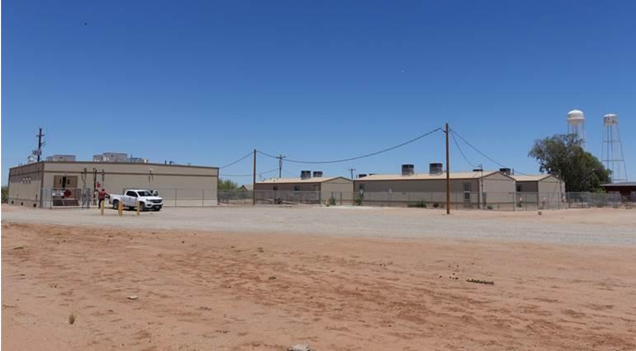
Santa Rosa Ranch School temporary modular units currently in use, until BIE completes replacement/renovation of original buildings.
