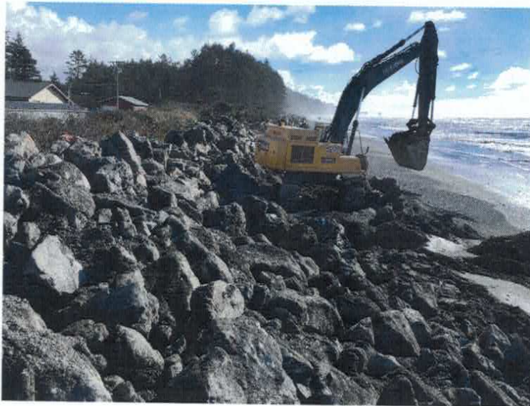
Building the temporary break wall
