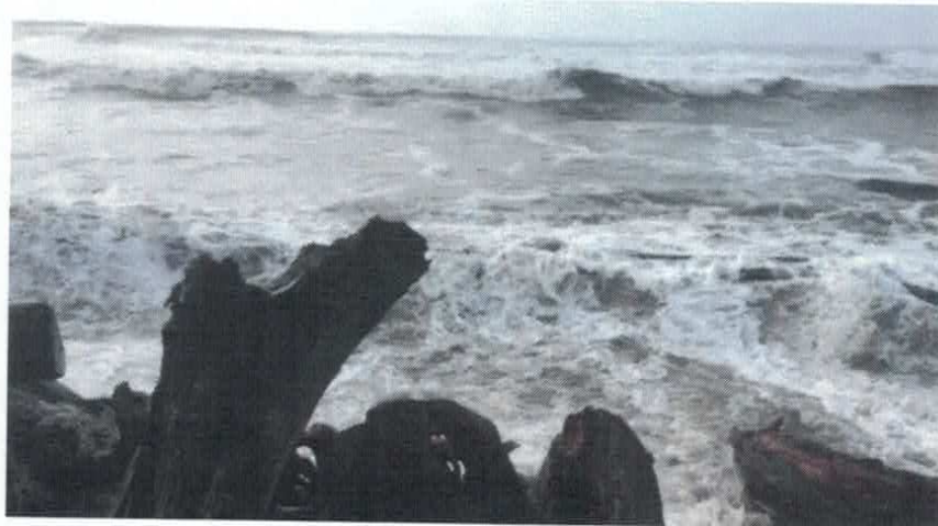
Pacific Ocean encroaching upon the temporary break wall
