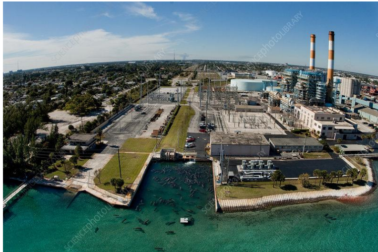
Figure 2. Manatees gathering around a Florida power plant Source: Science Photo Library.
