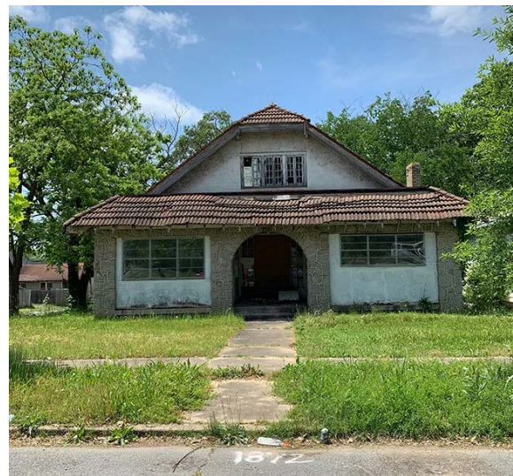
The Scipio Jones House, located in Little Rock, Arkansas, has fallen into significant disrepair. Source: Preserve Arkansas, 2022.
