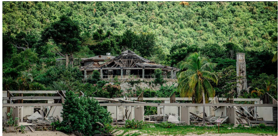
Caneel Bay in the U.S. Virgin Islands National Park, which requires significant capital investment to repair previous hurricane damage. Source: New York Times, 2020.
