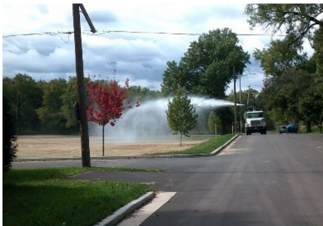
Restoring a remediated property at the DePue site.
