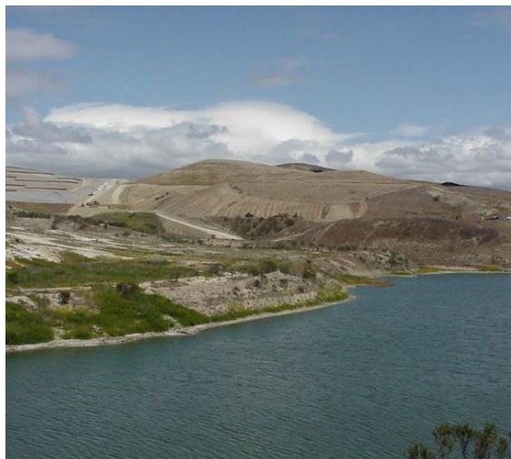
Three capped landfills and on-site runoff control facility pond.
