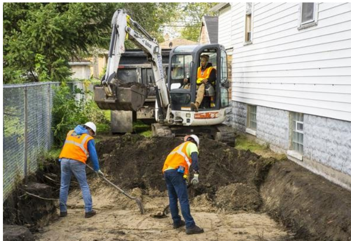
Excavating lead contaminated soil at the USS Lead site.
