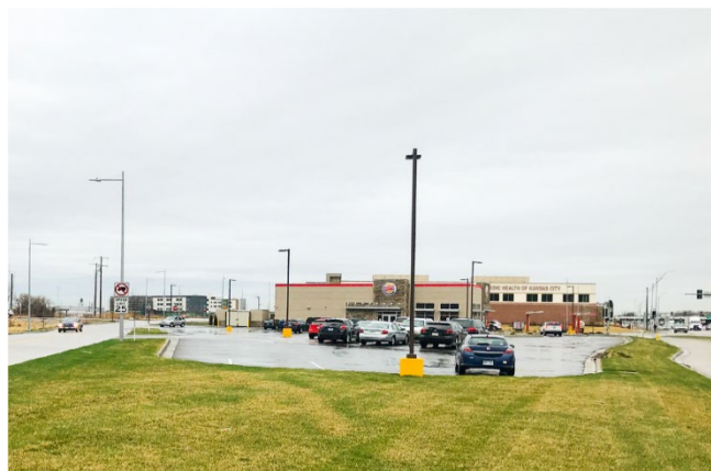
Armour Road Site After Cleanup
