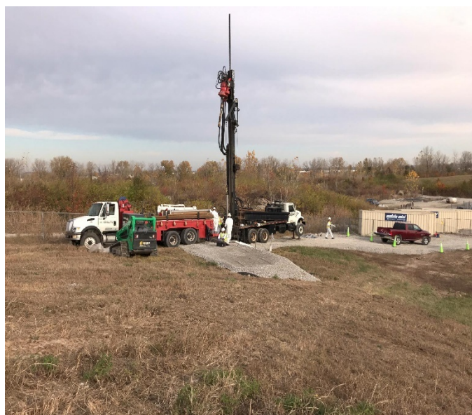
Boring installation at the West Lake Landfill site.
