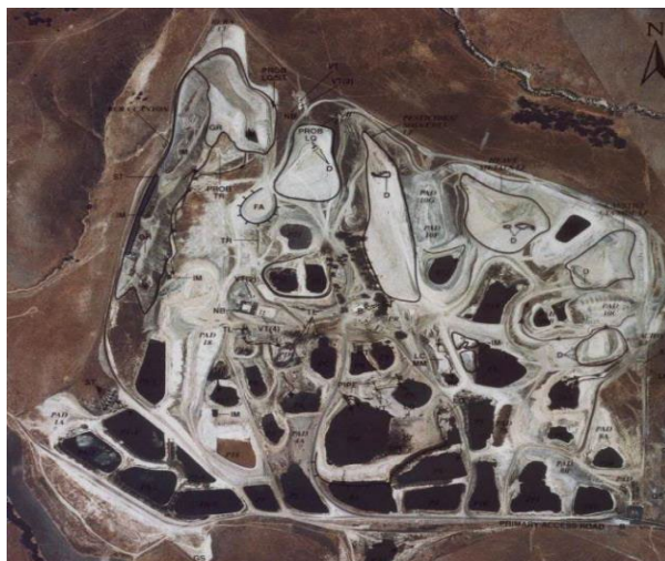
Aerial photo (1984) shows historic Casmalia site layout.
