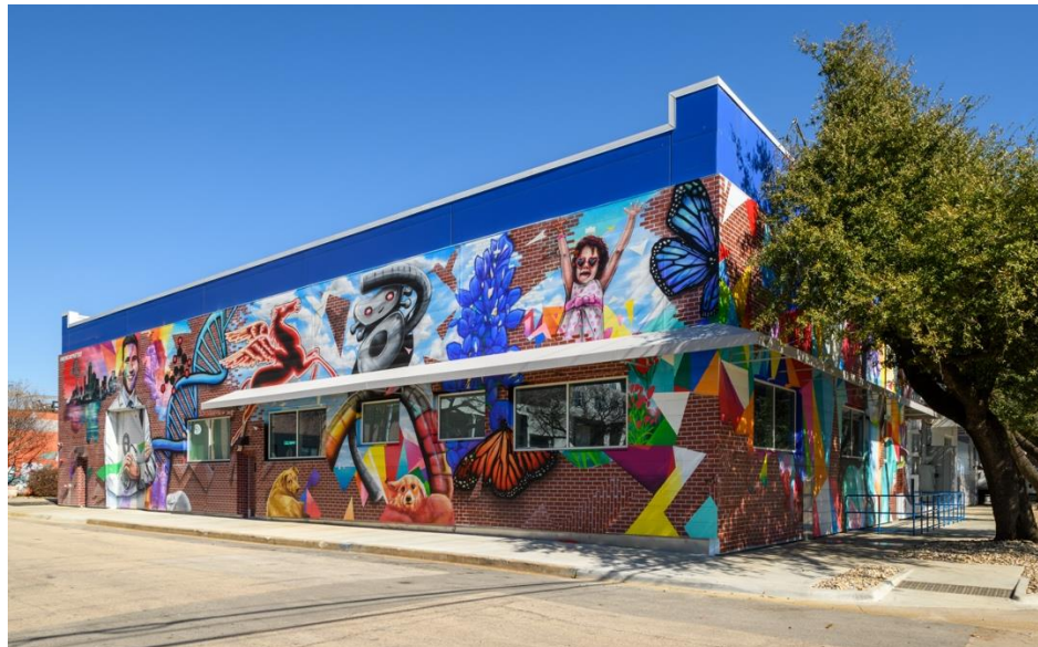
Image of MCCPDC Manufacturing Facility Exterior
