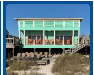
Structure elevation to mitigate flood damage
