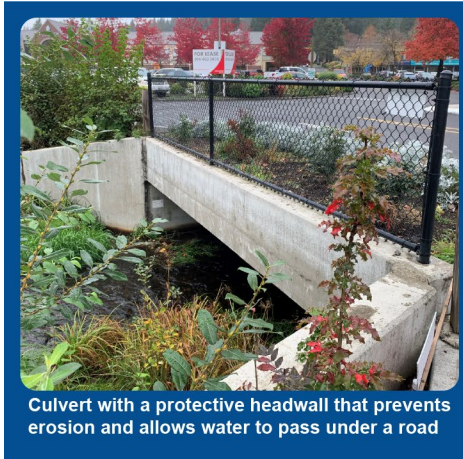
Figure 2: Examples of Hazard Mitigation Projects
