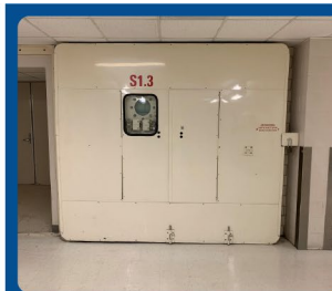
Watertight enclosure to prevent floodwater damage
