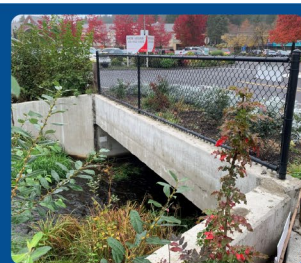
Culvert with a protective headwall that prevents erosion and allows water to pass under a road
