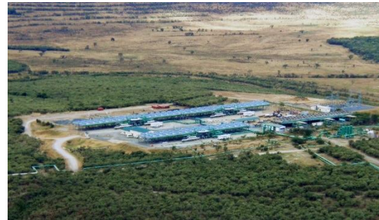
Olkaria geothermal power plant, Kenya
