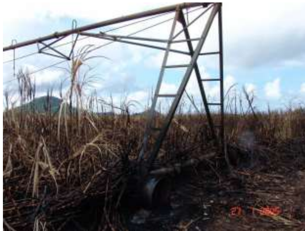
A wantonly destroyed centre pivot irrigation system on a former commercial farm Photo courtesy Farmer's Weekly magazine (SA)
