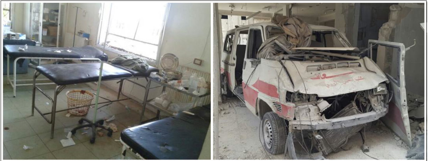
Figure 1: Damage to Health Facilities in Syria after Aerial Attack, Tel Shehab, Dara'a Province (left) and Al Khaf, Rural Damascus (right)
