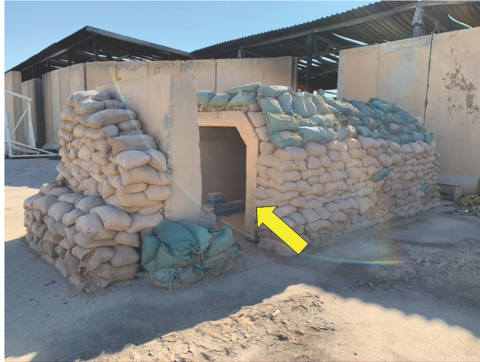
Above-ground indirect-fire shelter at Al-Asad Air Base damaged in the January 8, 2020 missile attack. Which lacked a protective door and offered limited protection from nearby blast impacts.
