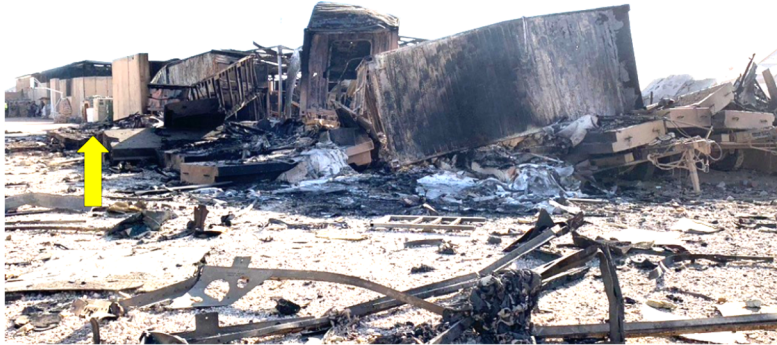
Damage to barracks and operations facilities at Al-Asad Air Base following the January 8, 2020 Iranian missile attack. Arrow indicates the indirect-fire shelter where Lt. Col. Johnson was located, approximately 60 feet from the impact site.
