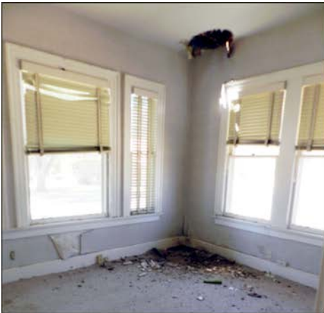
Interior damage of Kerrville Medical Center.
