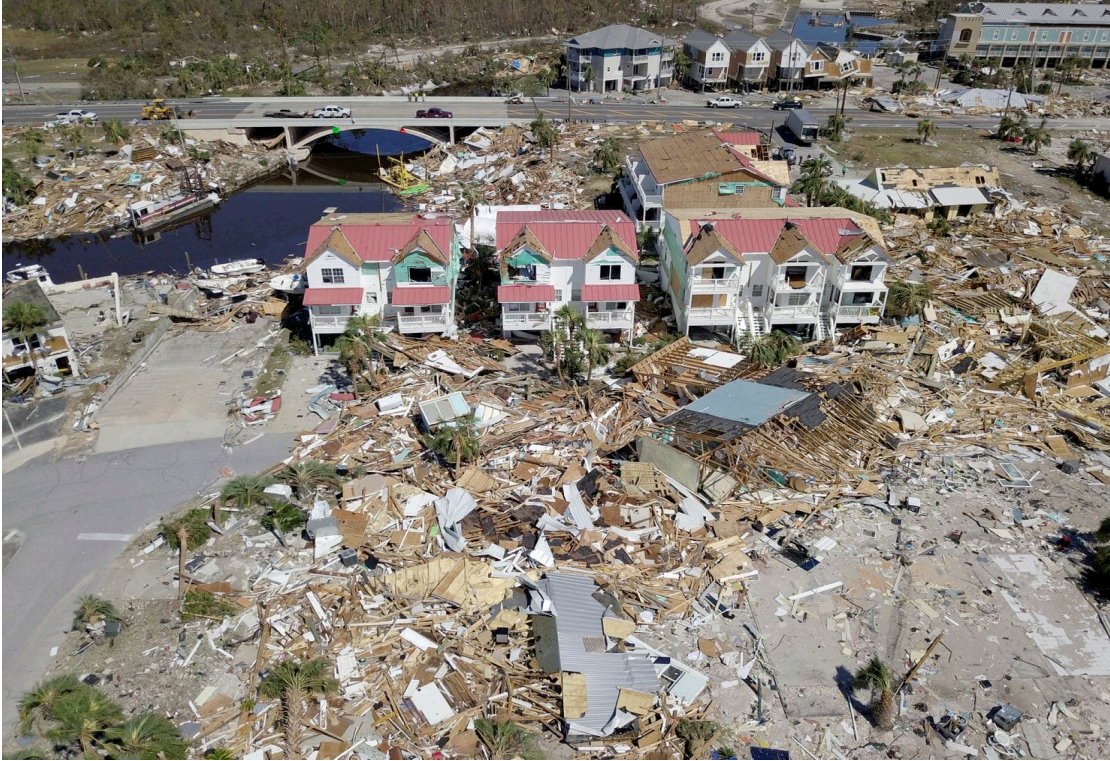
Figure 3: Mexico Beach, FL after Hurricane Michael (2018). Older homes not built to code are completely destroyed. But newer homes built to code suffered relatively minor damage. (Dronebase/Reuters, Handout/Reuters).
