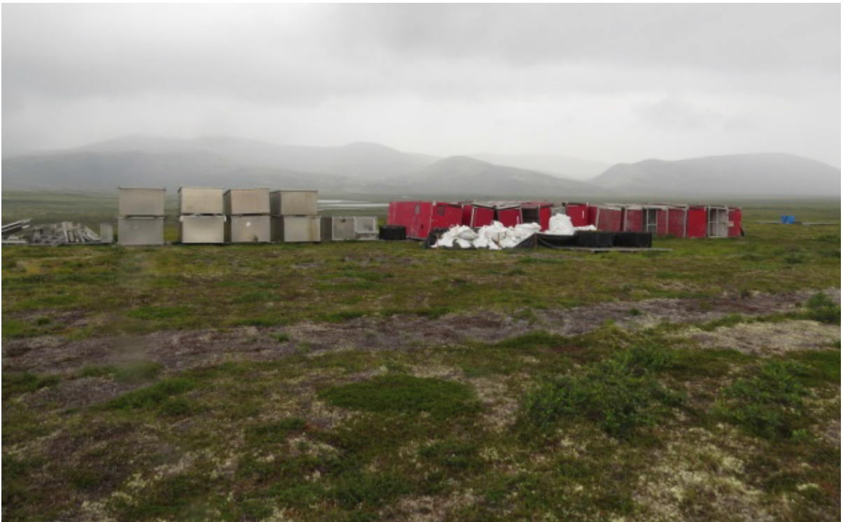
Photo: Alaska DNR July 2015. Boxes for line heaters
