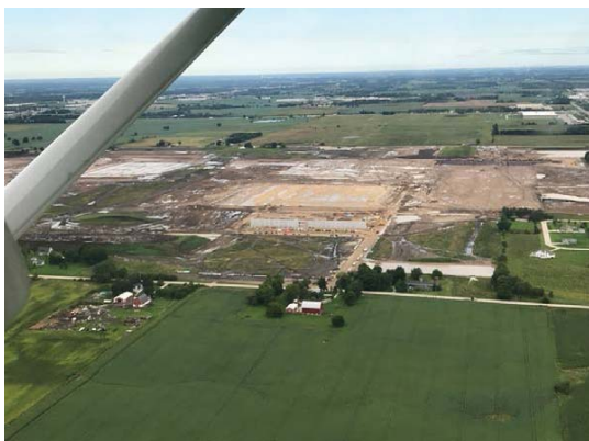
Foxconn Phase 1 Construction Site – September 6, 2018
