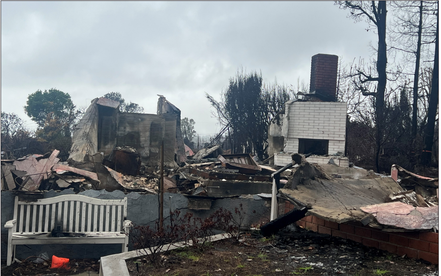
Figure 4: Fire Damage Following the Palisades Fire Los Angeles, California
