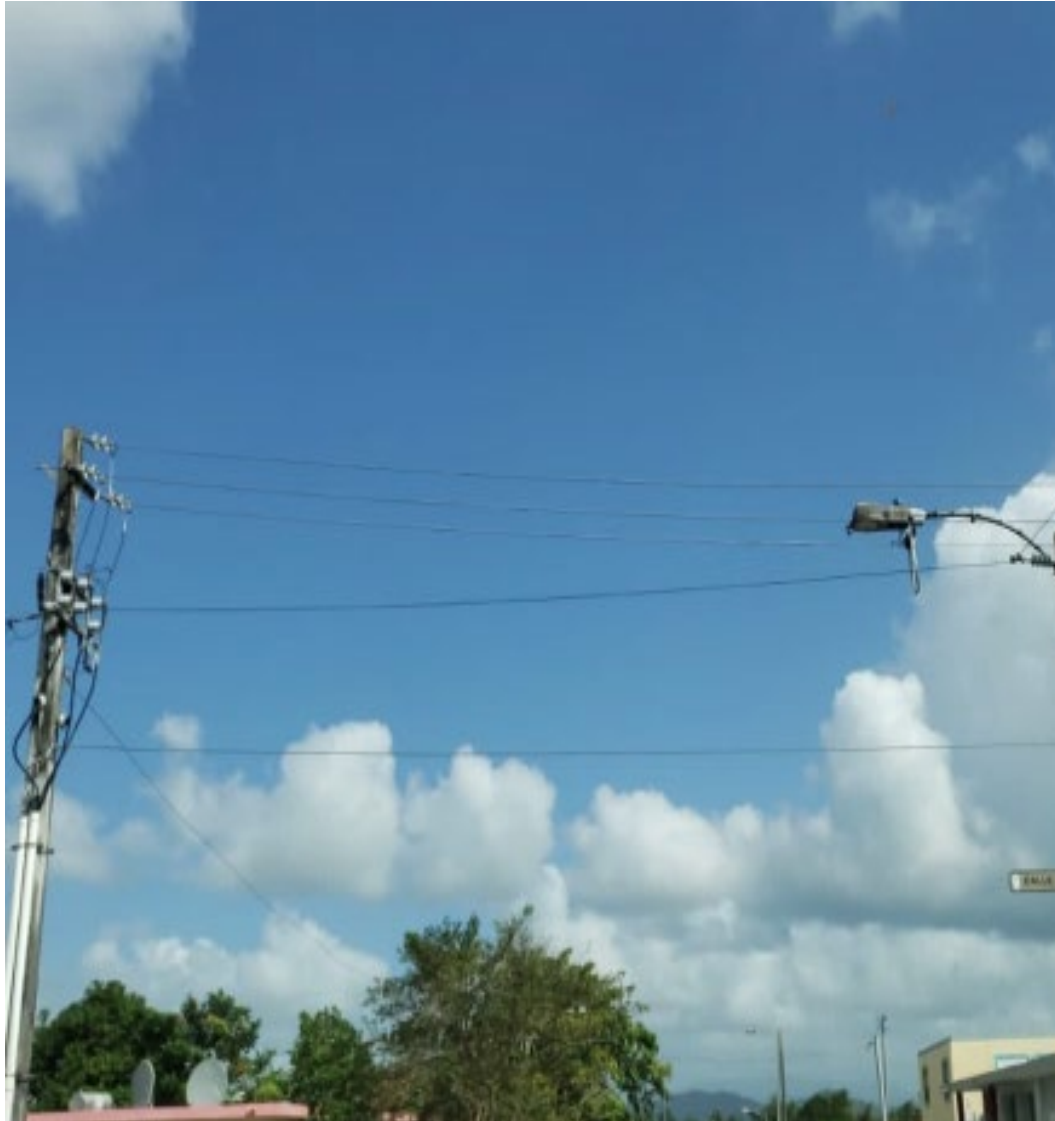
Primary wire ended on street light pole within limits of approach to primary line.
