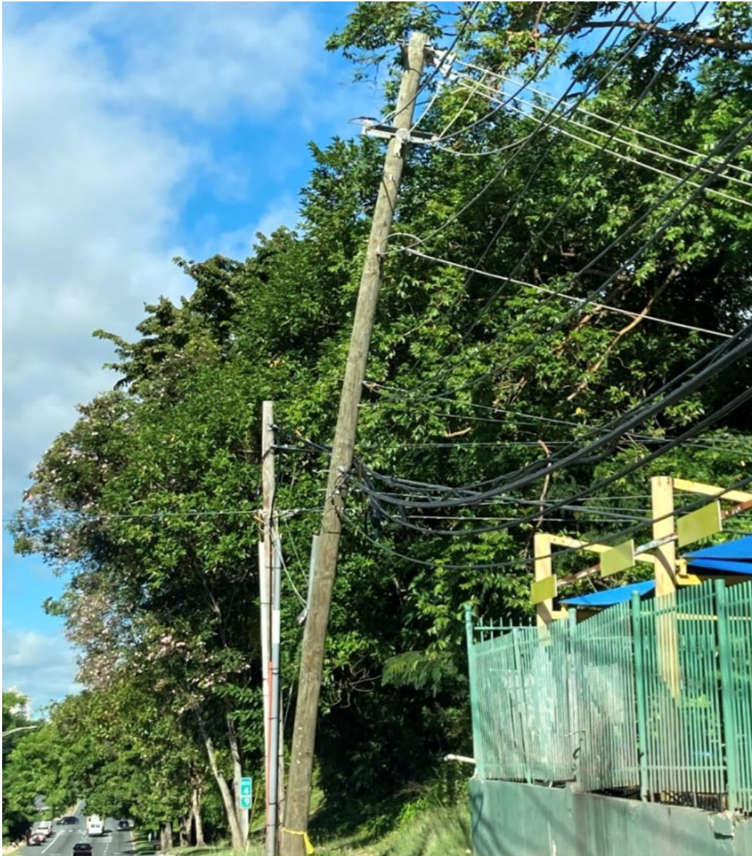
New pole installed incorrectly.
