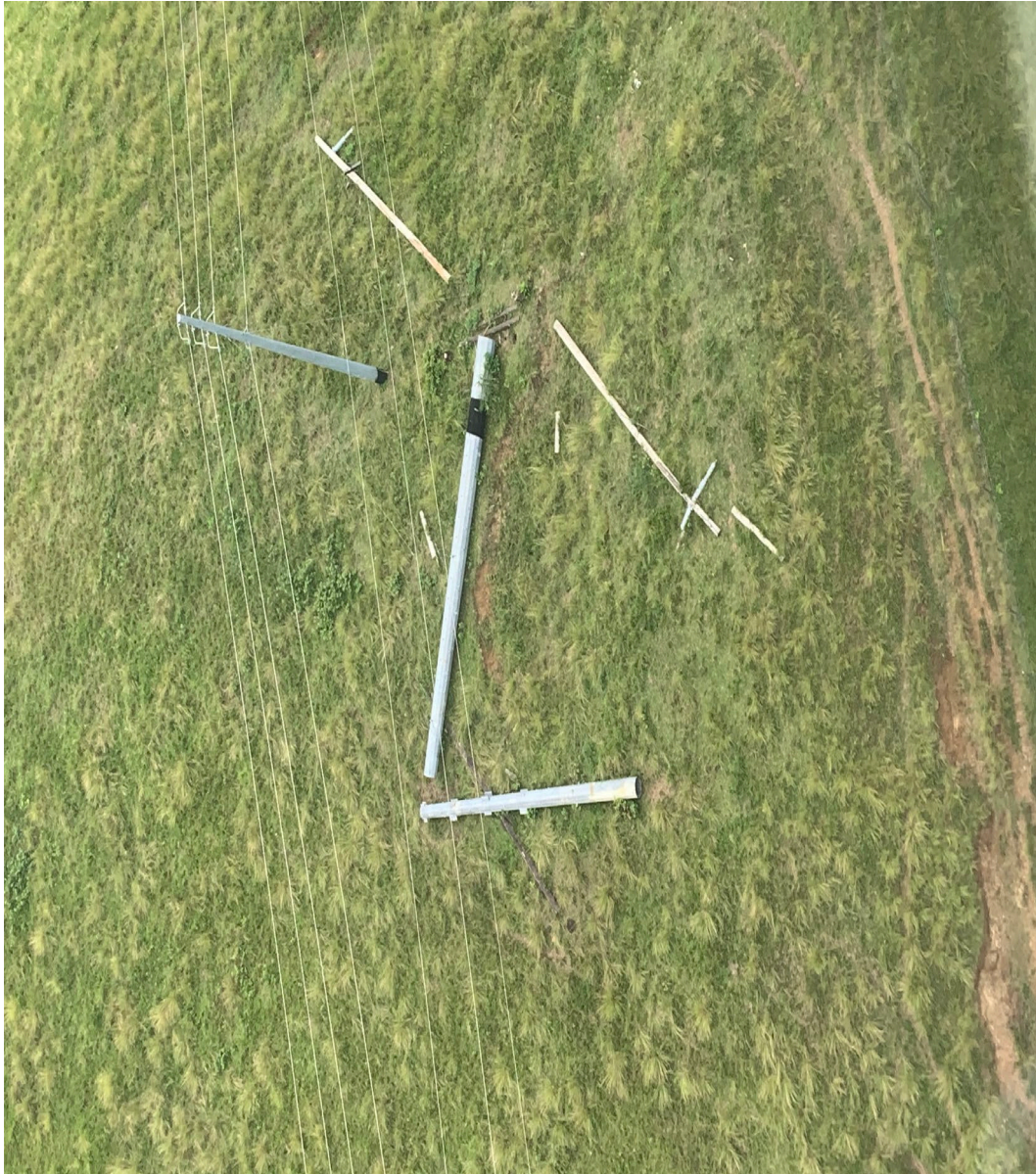
Failed Tx pole circuit.
