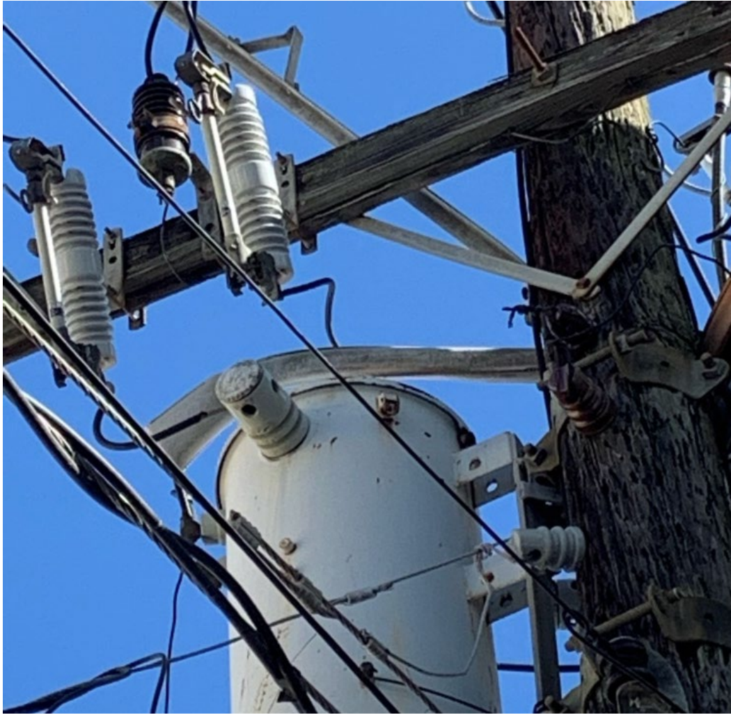
Primary conductor laying on top of transformer with line hose bleached white from sun exposure.
