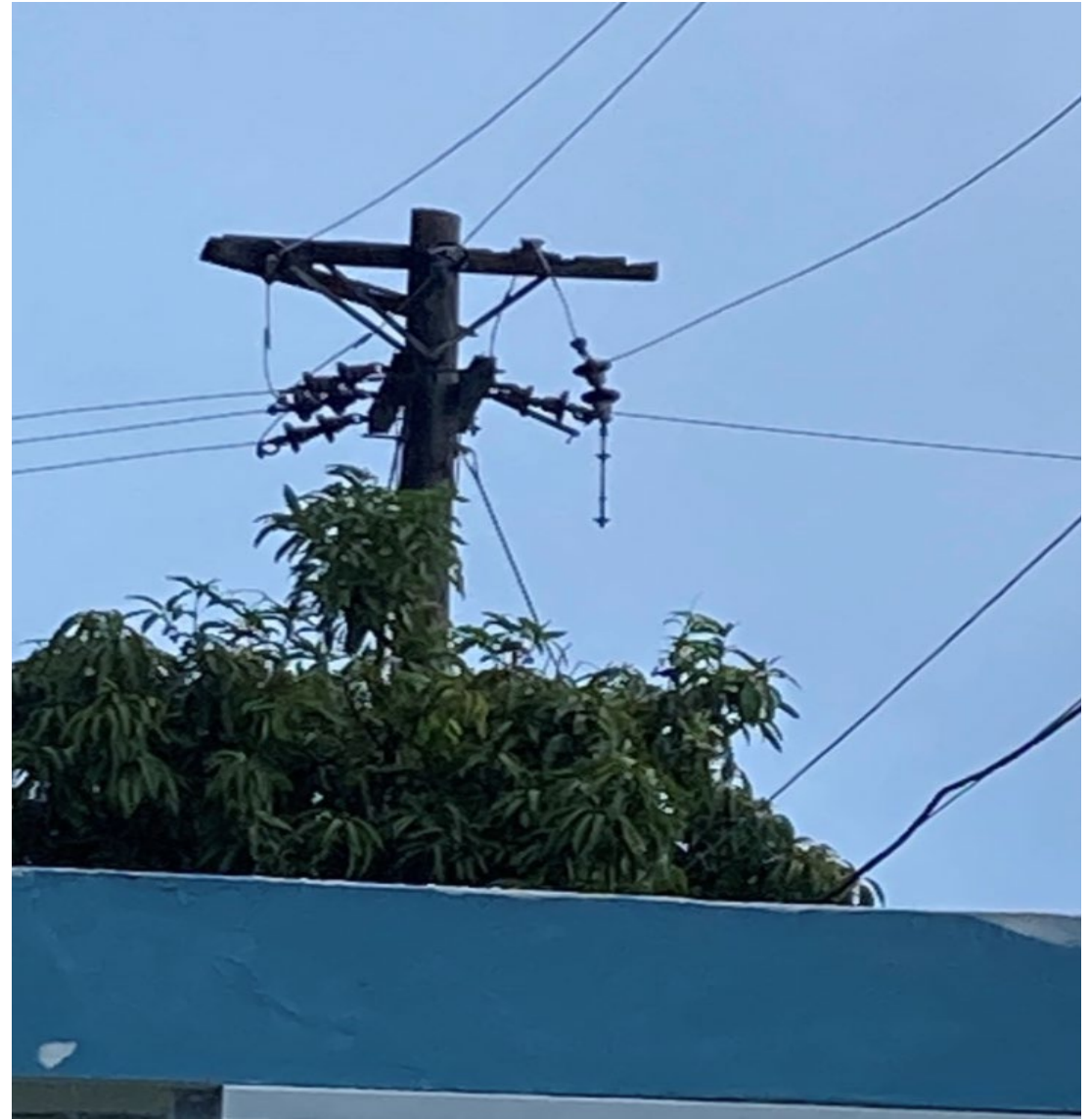
Failed cross arm. Failed hardware. Primary laying in cross arm.
