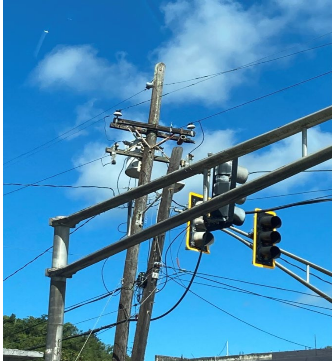
Hardware failure, wire against pole.
