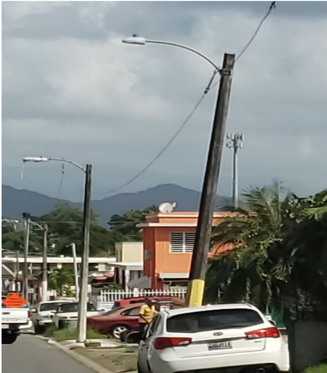
Primary wire suspended from streetlights.
