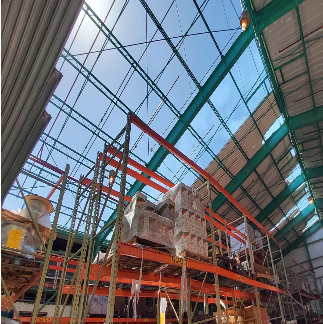
Aguirre Power Plant Warehouse. Roof missing since Maria, not prioritized causing heavy damage to material and racking from repeated rainfall.
