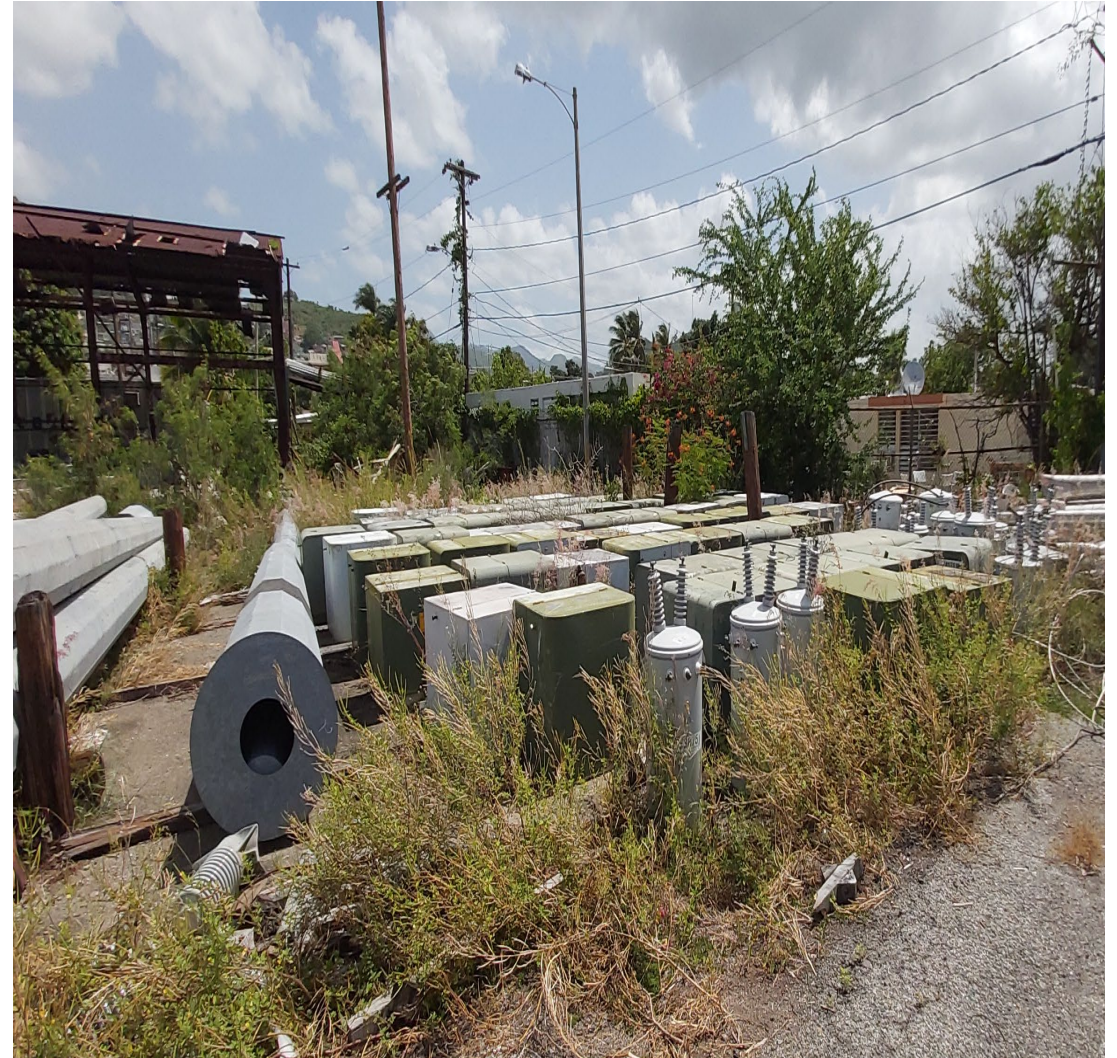
Yauco Yard. Non-stock Padmount Transformers 10+ years old.
