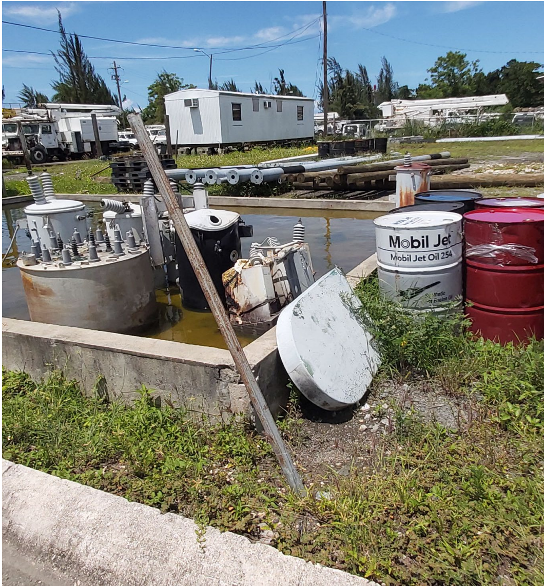
Palo Seco Transmission Warehouse Yard - Secondary Oil Containment about to overflow. Pre-LUMA System and Facility Conditions
