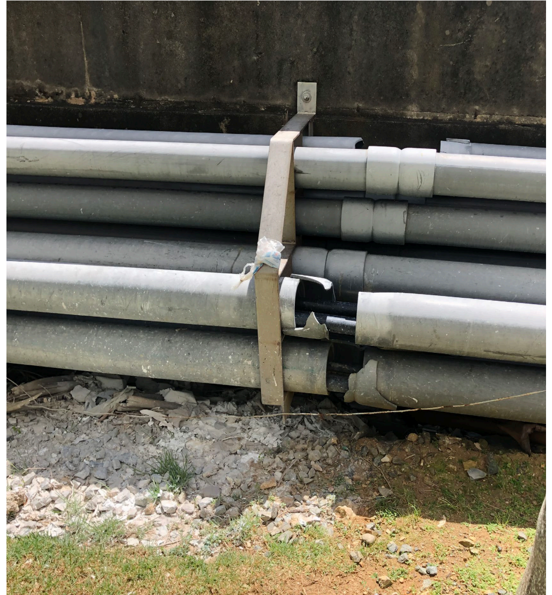
Failed primary underground cable.
