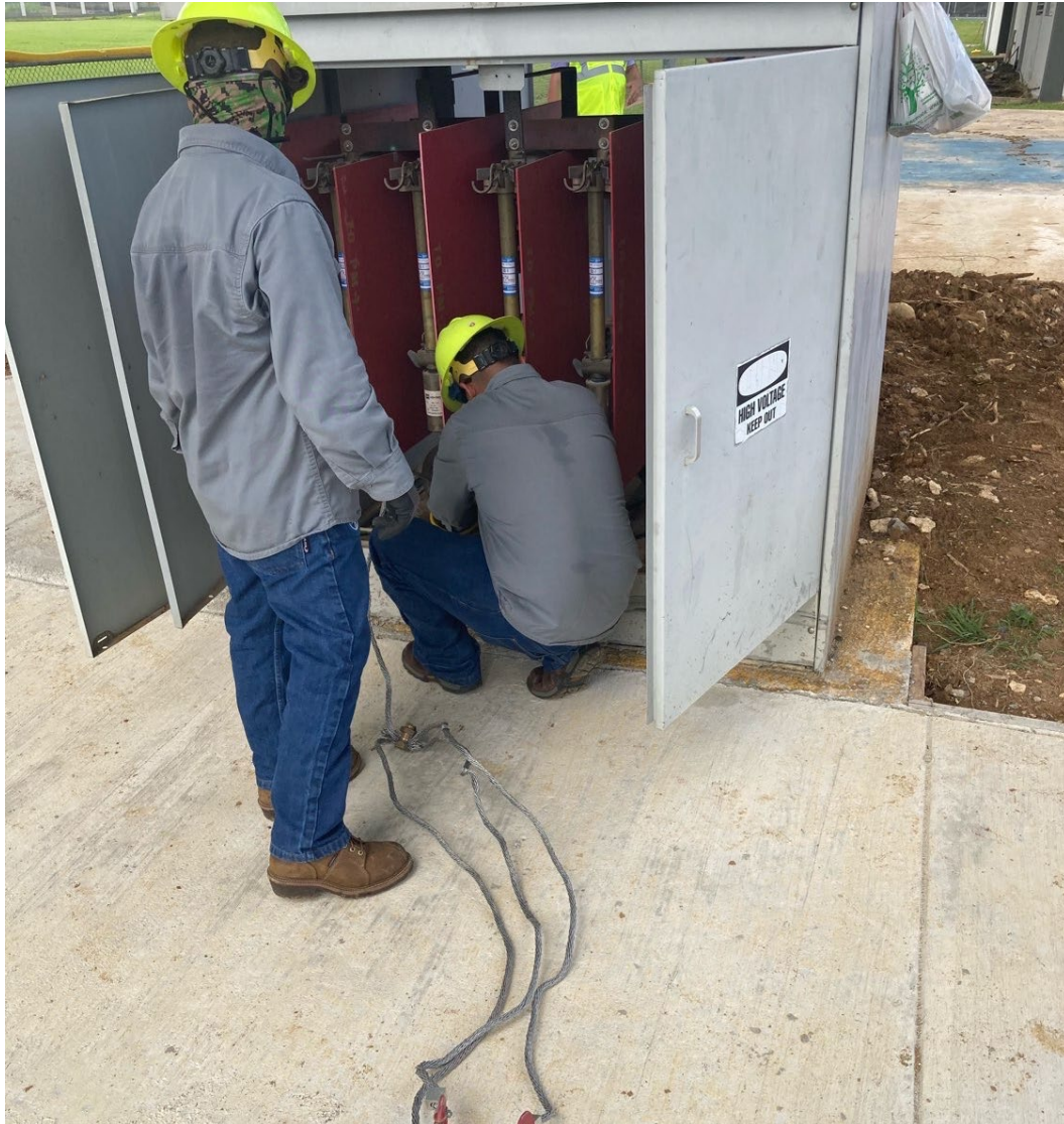
The phases were contacting each other, rubber coverup installed instead of repairing.
