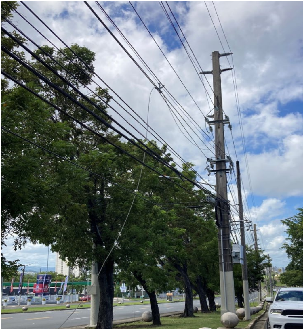
Damaged neutral conductor.
