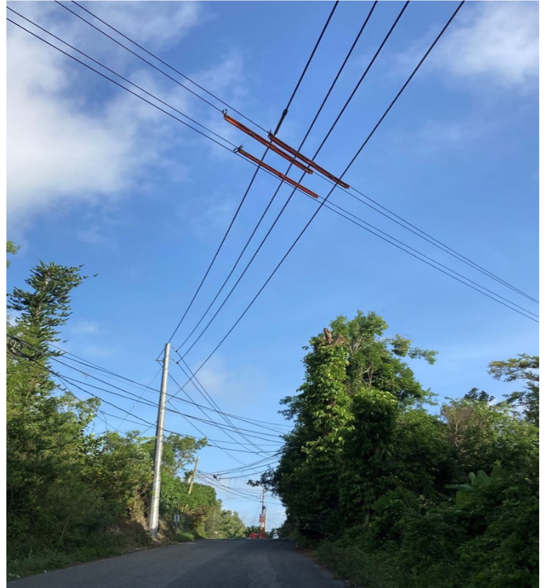
Circuit against circuit. Line hose installed to separated not expectable.
