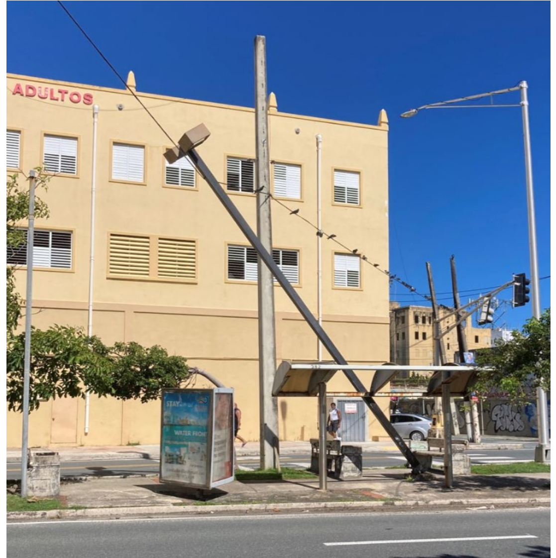
Failed streetlight pole on telecommunication cable.
