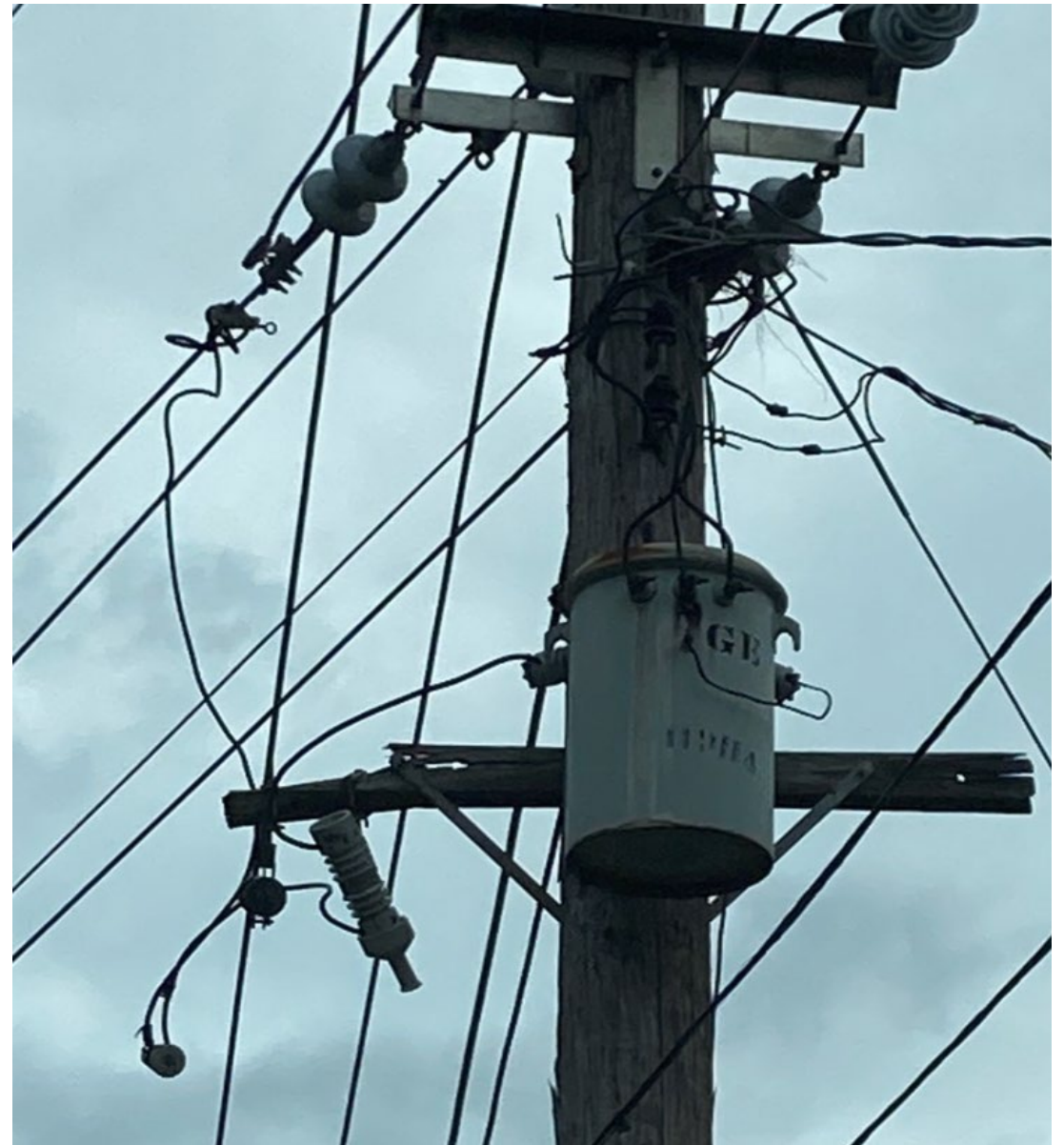
Failed cross arm. Poor workmanship.
