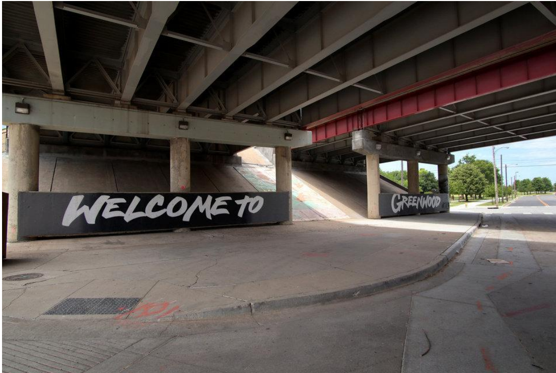
I-244 Underpass Was Intentionally Placed Through Greenwood to Destroy the Remaining Remnants of the Greenwood Community
