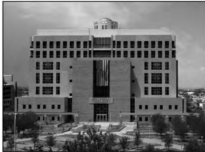
COMPLETED LANDSCAPE PROJECT, JULY 4, 2013
