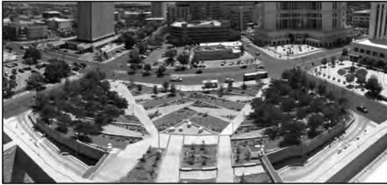
COMPLETED LANDSCAPE PROJECT, TOP VIEW, 2014
