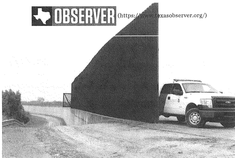
In Hidalgo County, about 20 miles of wall already exist. GUS BOVA
