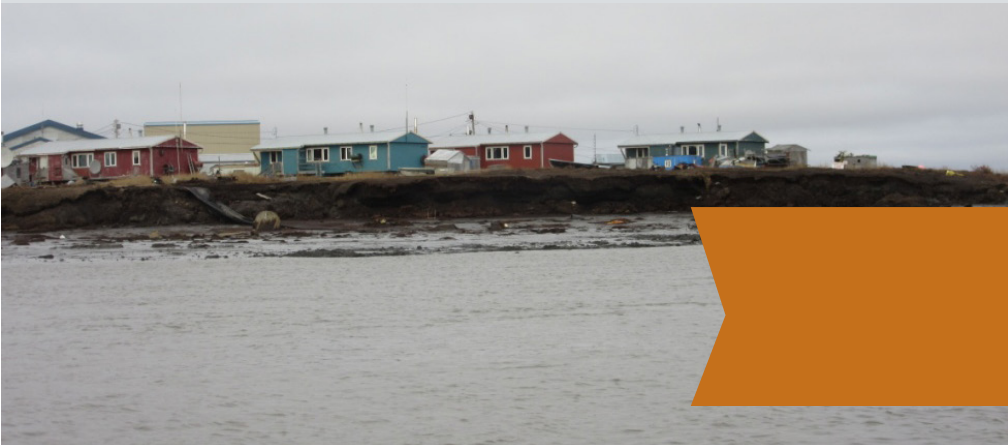
Barge Landing Destroyed in 2005
