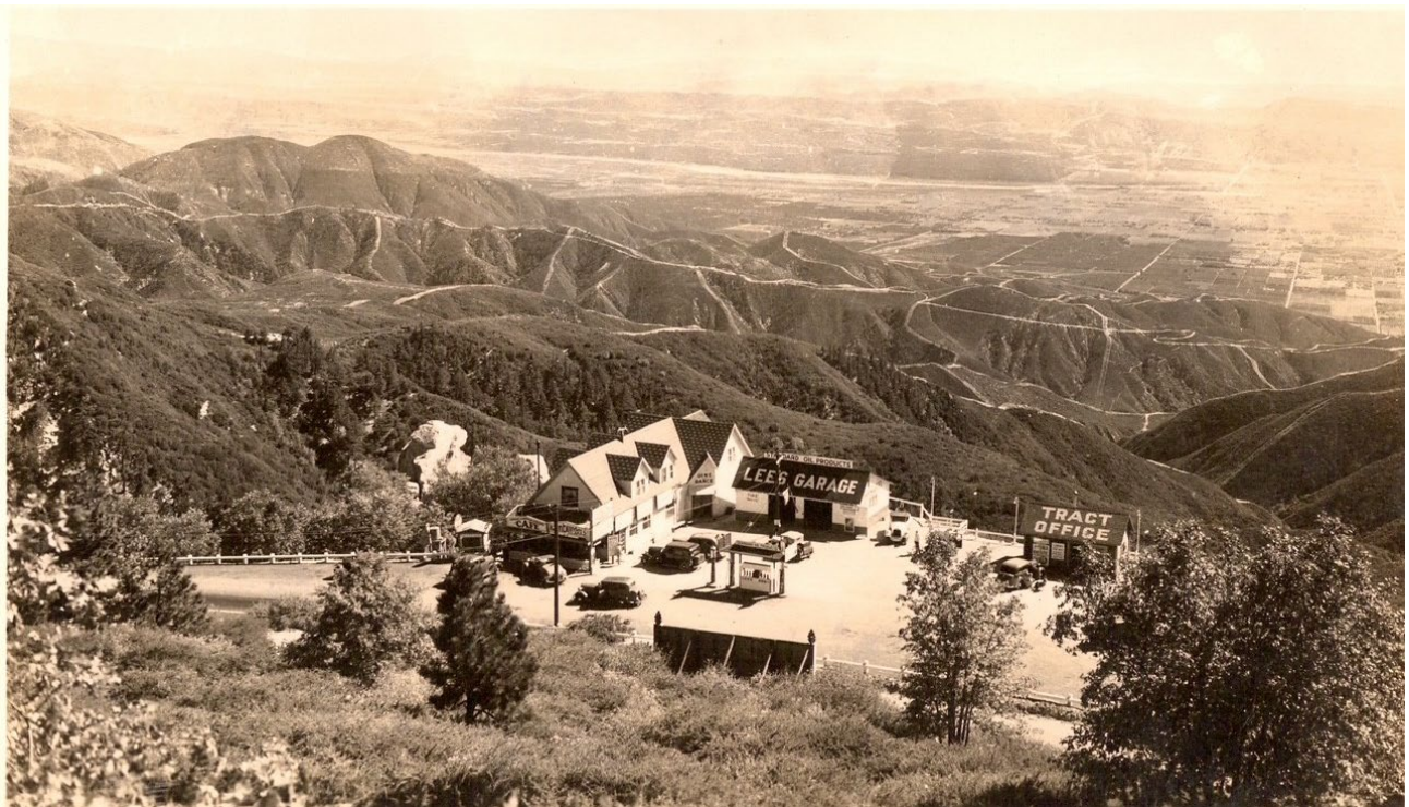
Figure 1. A view of the San Bernardino National Forest from the 1930’s showing robust fuel breaks and access roads.
