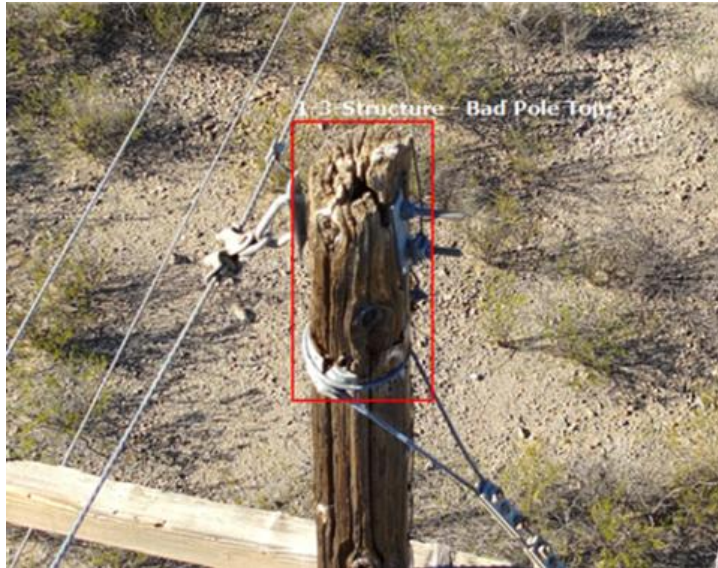
Structural aging of poles, Fairbank, AZ
