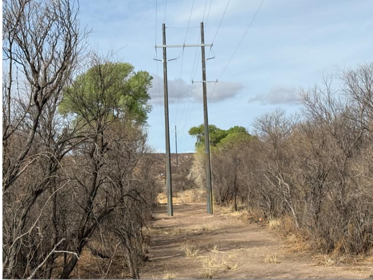
Completed Fairbank project
