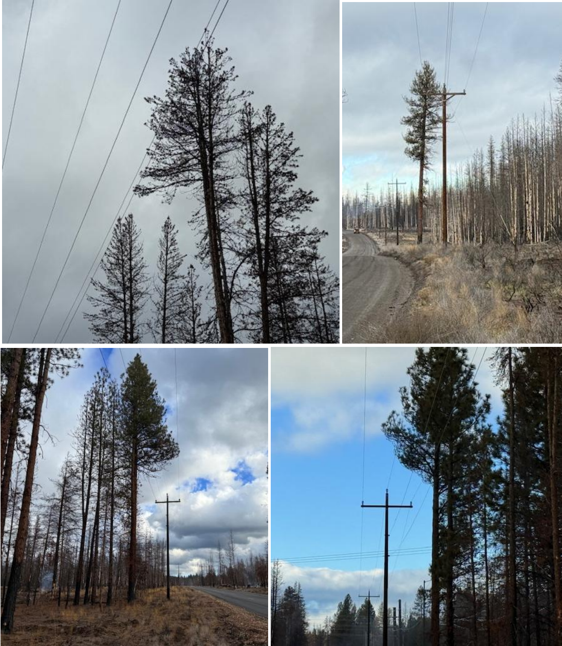
Hazard trees unaccounted for by USFS following the Darlene 3 Fire
