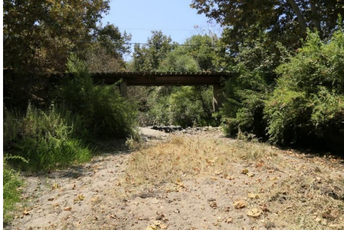
Image 3: Dry South Fork of the Tule River.
