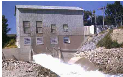
Figure 3: The Pilot Butte Power Plant Source: Bureau of Reclamation
