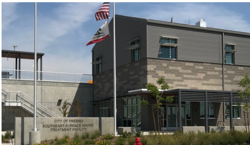
The recently completed City of Fresno Southeast Surface Water Treatment Facility is actively contributing to meeting the water usage consideration goals of the Blueprint.
