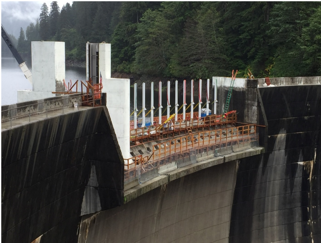
Gate Piers Complete – Flashboard Columns Erected
