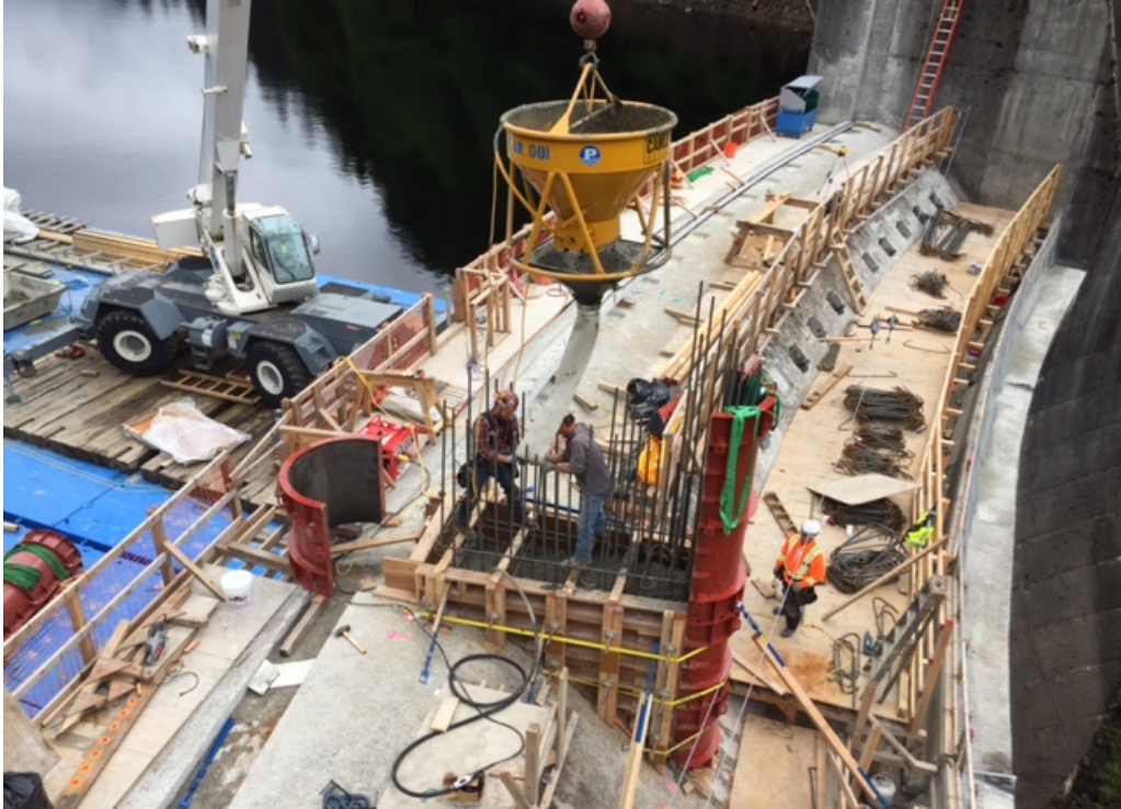
Middle Pier Concrete Placement
