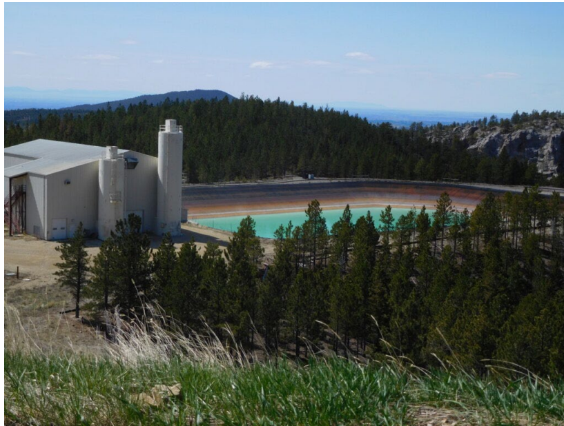
One of two water treatment plants constructed to neutralize acidic water draining from the mine. Because there is no way to stop the exposed rock from generating acidic runoff, mitigation must continue around the clock and “in perpetuity.” Photo by Paul Boyer
