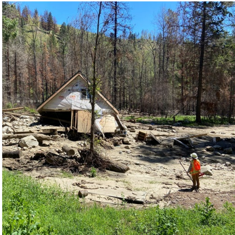
Figure 3. (above) A cabin that was destroyed in 2022 following a post-fire debris flow from an upslope wildfire burn scar.
