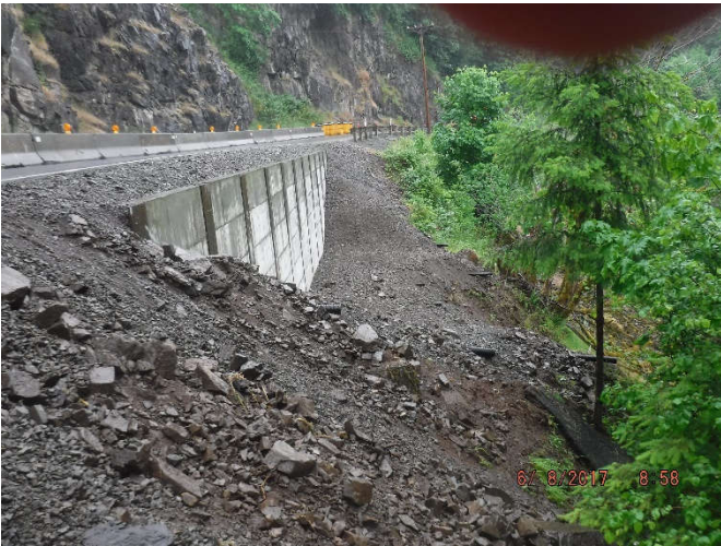
Soldier pile retaining wall
