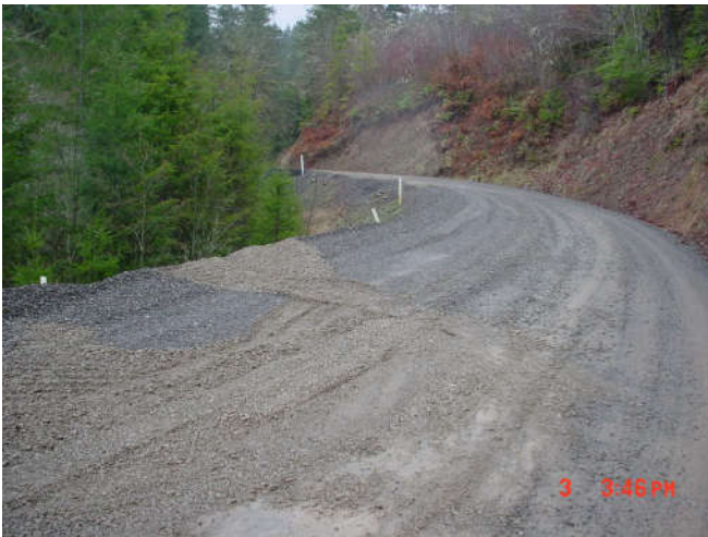
Section of roadway that is maintained as gravel
