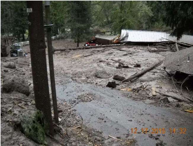
Home and roadway damaged by a slide
