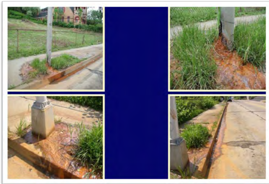
Figure 4. AMD emanating from lamp posts in front of the John Wesley AME Zion Church
