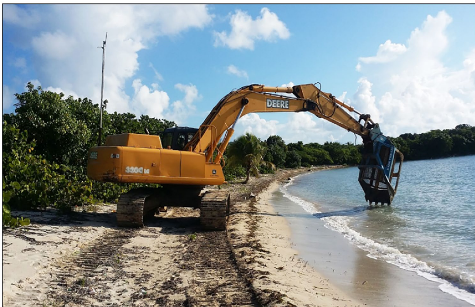
Figure 10: Remotely Operated Excavator Used at Cleanup Sites on Vieques, Puerto Rico
