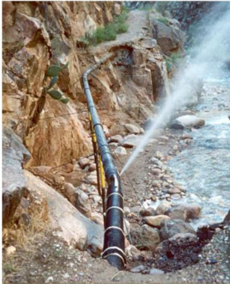
Pipeline – Grand Canyon National Park
