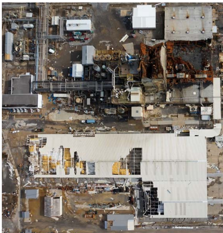
Aerial image from CSB of the Bio-Lab facility in Westlake, LA, in the aftermath of Hurricane Laura and the chemical fire and release. Source: U.S. Chemical Safety and Hazard Investigation Board
