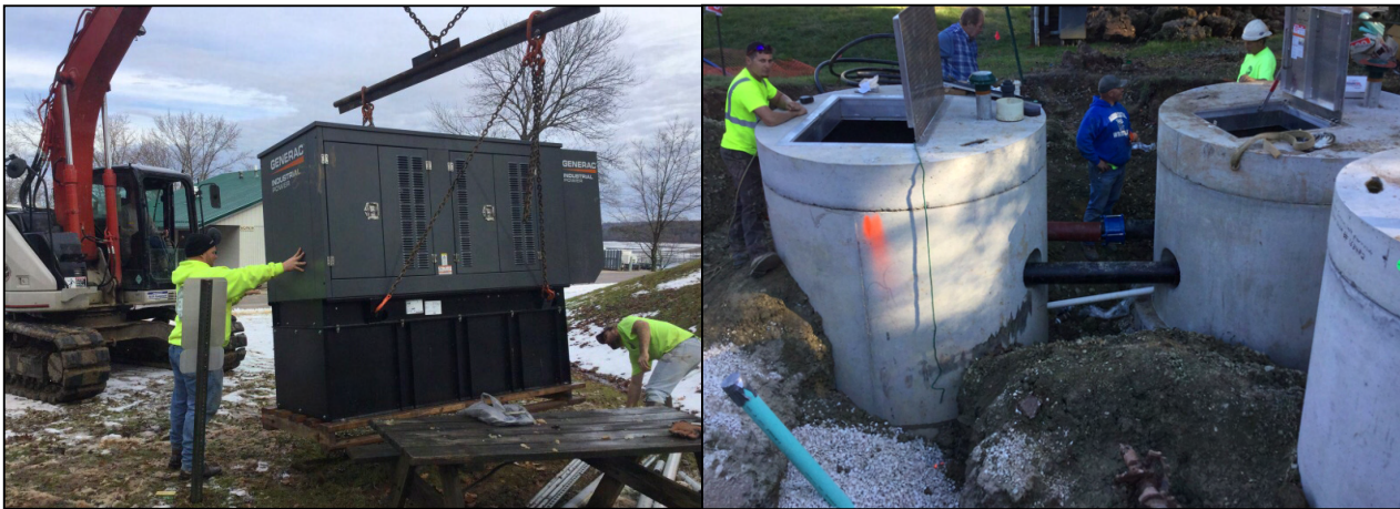
Sanitary sewer improvements at Seneca.
