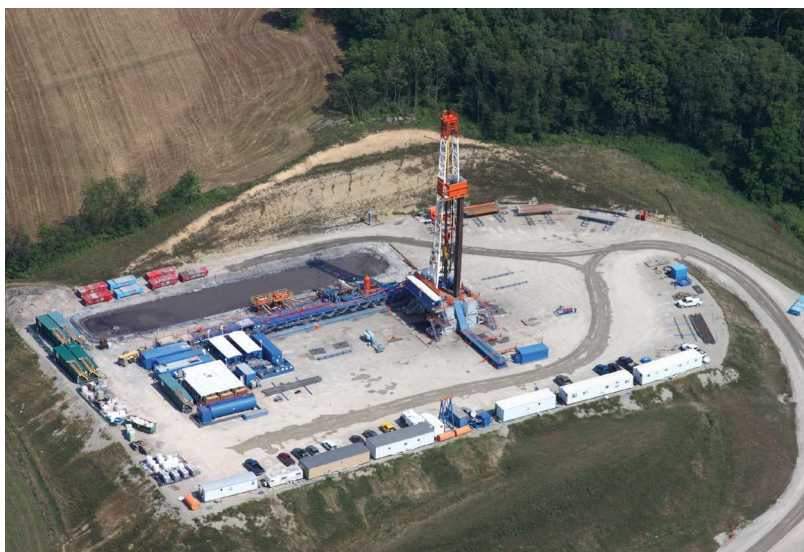
Marcellus-Shale gas drilling well in Southwestern Pennsylvania.
