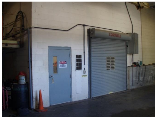
Secure Storage Room - Exterior
