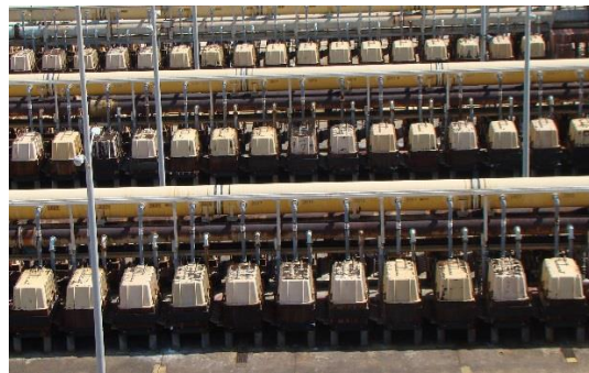
Electrolytic Cell "Circuit"
