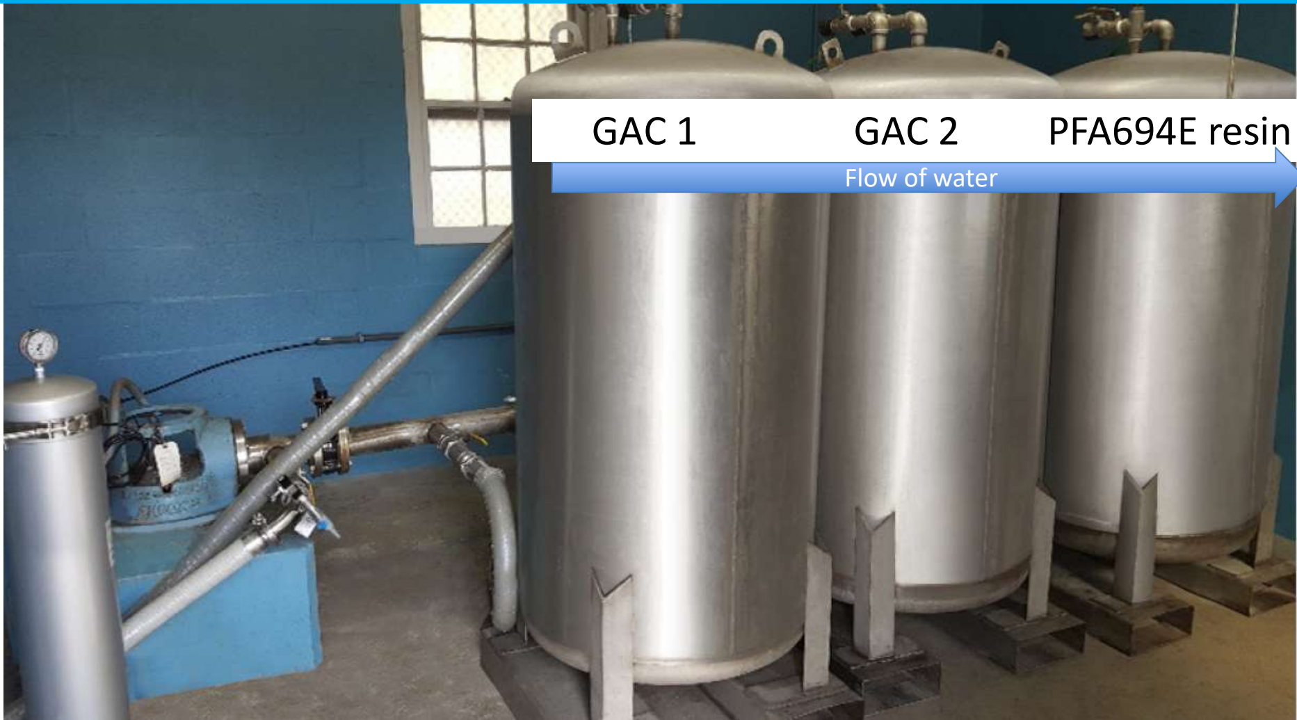
Photo courtesy Altair Equipment Well 10
