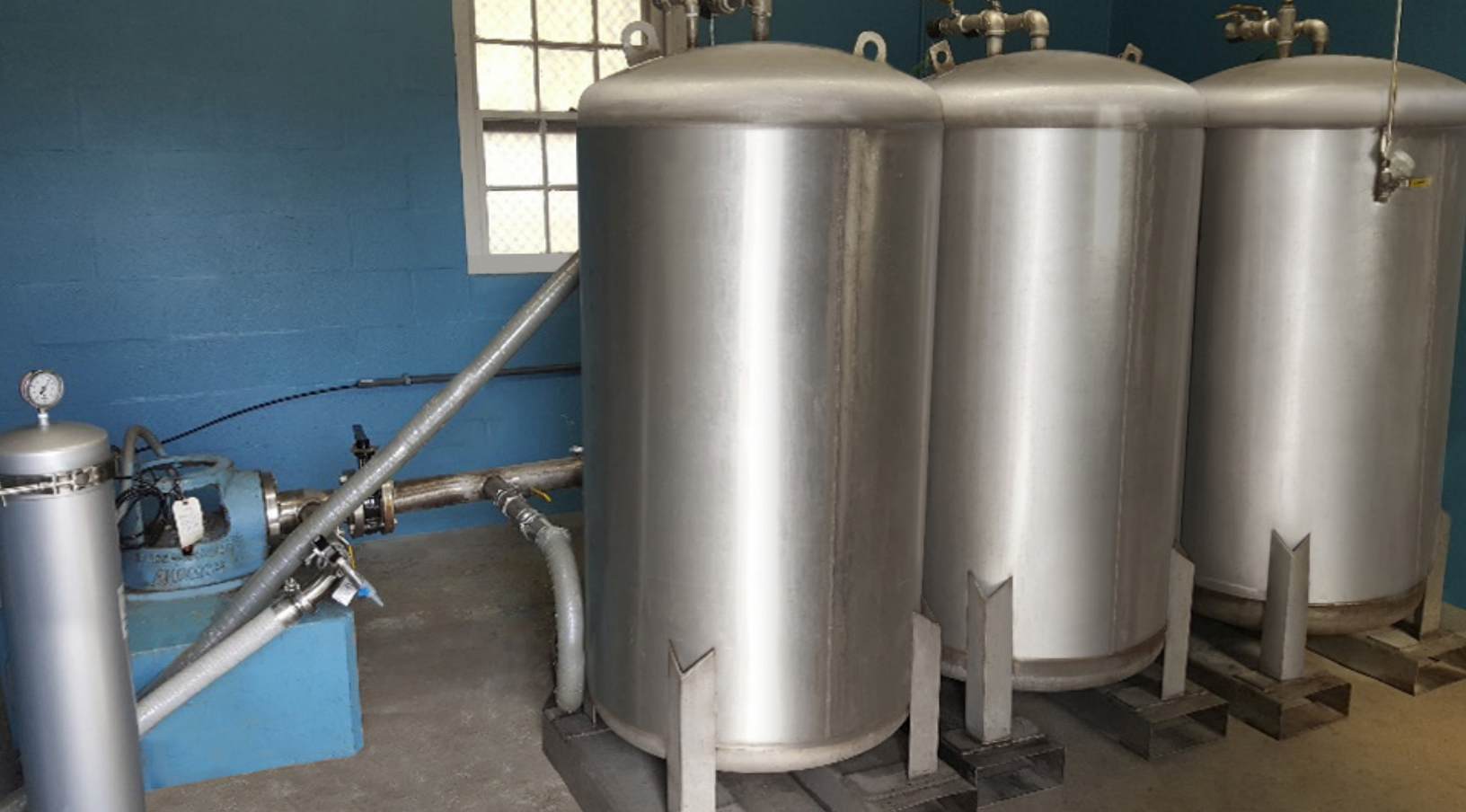
Horsham's lead-lag GAC and resin system (L to R) GAC, GAC, Resin.
