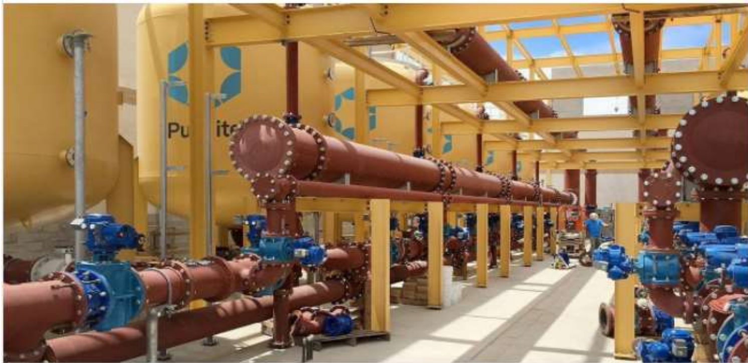
World's largest nitrate removal plant with 13,000 ft 3 of Purolite A520E resin
