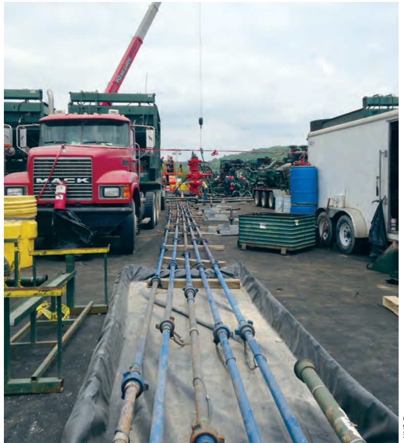
Completion equipment at a gas well.
