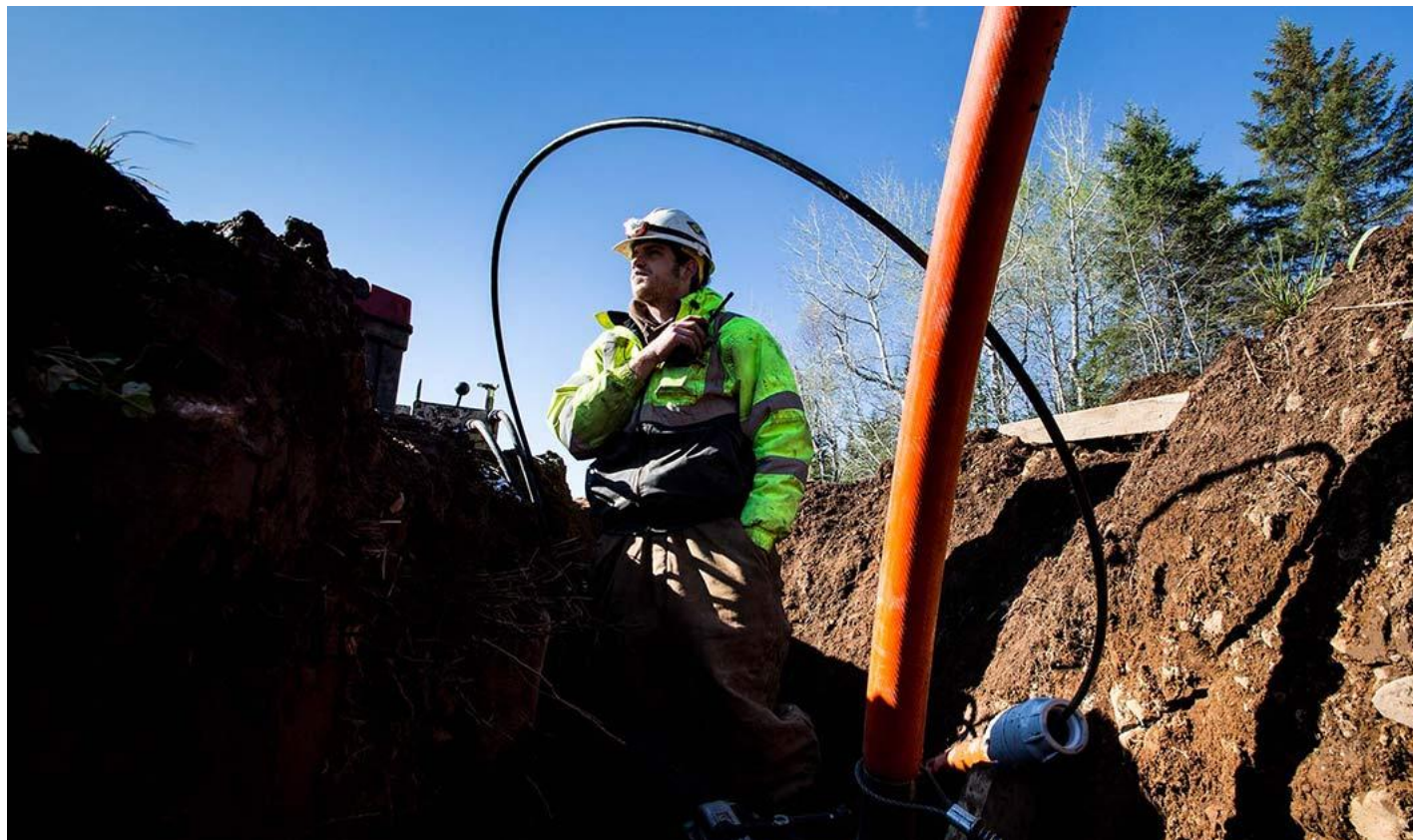
Bryant Hancock, a contractor for Lake Connections, buries fiber optic lines in May in rural Lake County, Minnesota. | M. Scott Mahaskey/Politico
