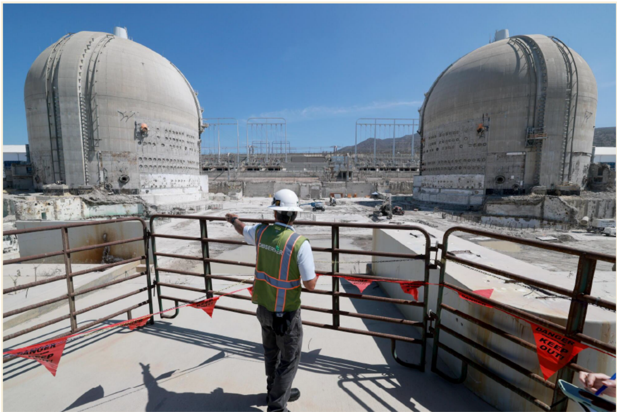
Kevin Sheek points to decommissioning work around reactor containment domes during a tour of the nuclear waste storage facility. (Allen J. Schaben / Los Angeles Times)
