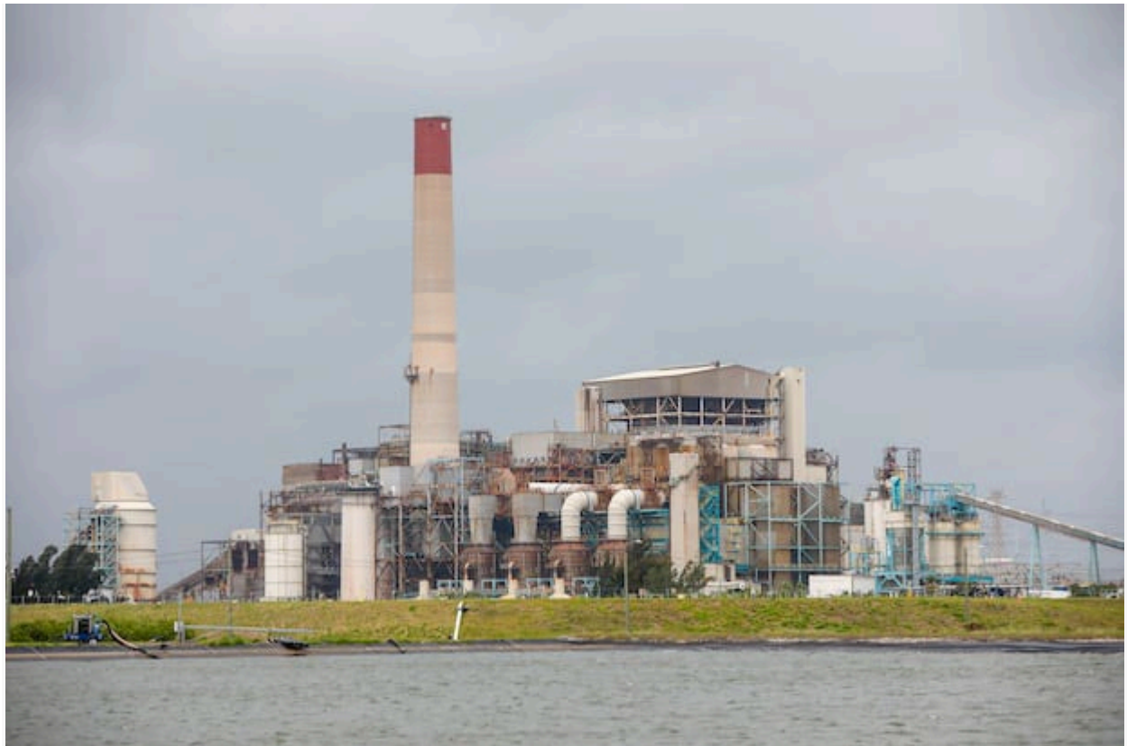
The power plant at the TECO Big Bend Power Station, which can use either natural gas or coal, on April 11 in Apollo Beach. [ JEFFEREE WOO | Times ]
