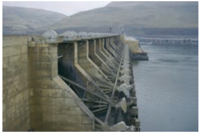
John Day Dam, Source: CRITFC
