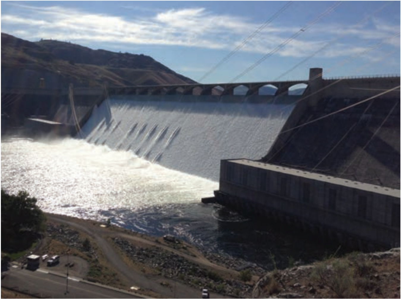
Grand Coulee Dam, Source: Keith Kutchins
