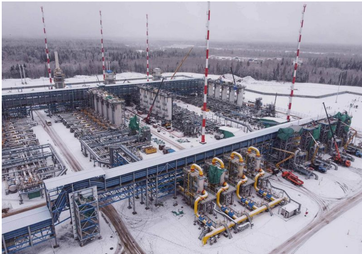
The starting point of the Nord Stream 2 pipeline in Ust-Luga, Russia. Photographer: Andrey Rudakov/Bloomberg
