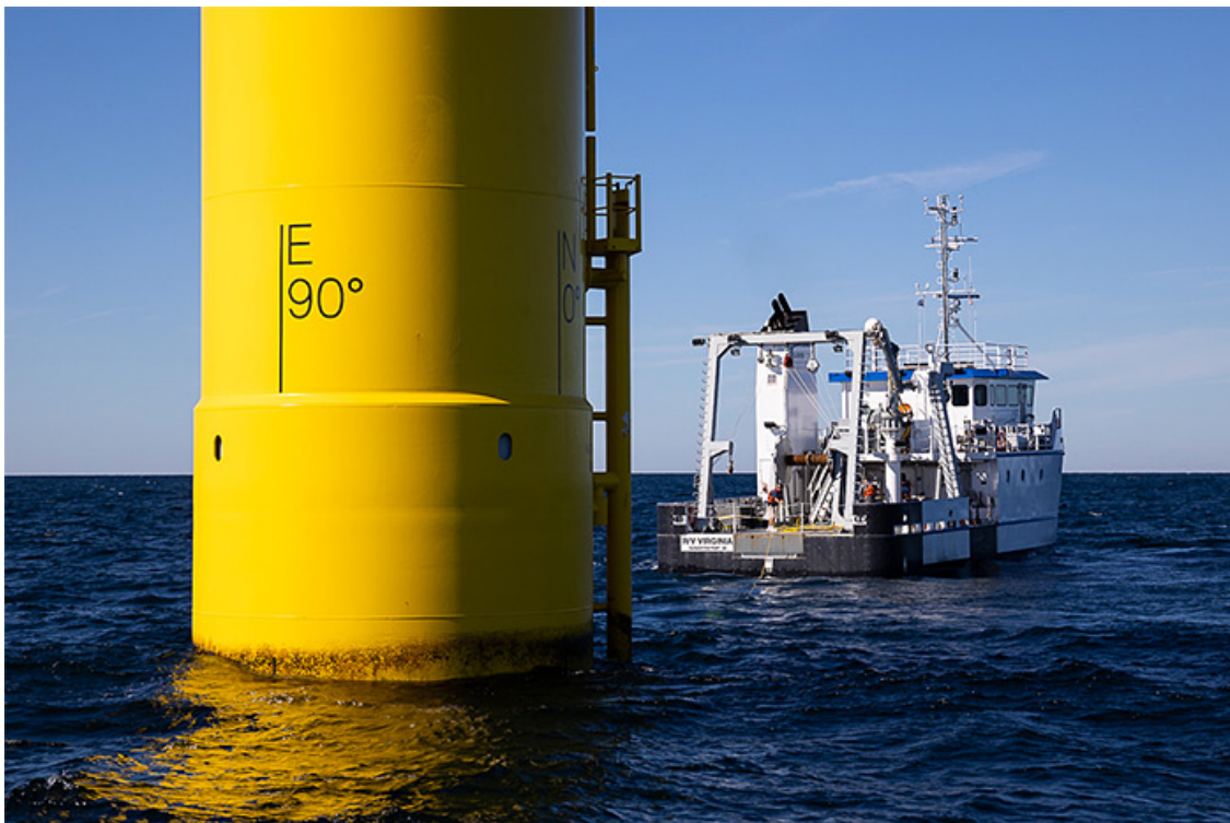
Dominion Energy's pilot offshore wind project off the coast of Virginia Beach. | Francis Chung/E&E News
