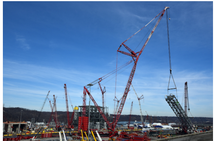
The scale of the project is unprecedented in the area, and uses one of the world's largest cranes at nearly 700 feet tall, it can lift 3,500 tons.
