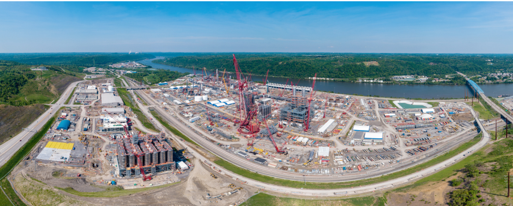
The Shell Pennsylvania Petrochemicals Complex near Pittsburgh will employ 1,000 electricians for more than a year, making it one of the largest projects in the IBEW.
