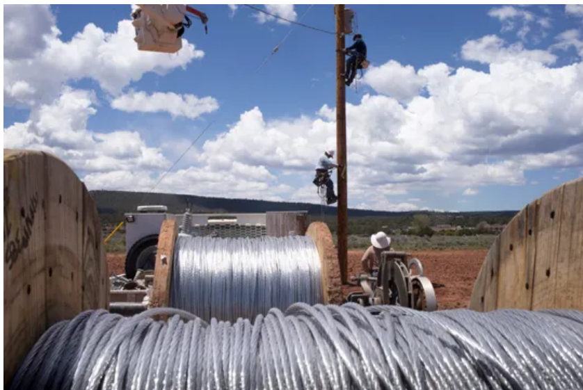
Tommy Skye (bottom) of the Navajo Tribal Utility Authority and Jake Haines of the Salt River Project work on a pole May 13, 2019, at the home of Ella and Herman Lynch in Oak Springs, on the Navajo Reservation. (Photo: Mark Henle/The Republic)
